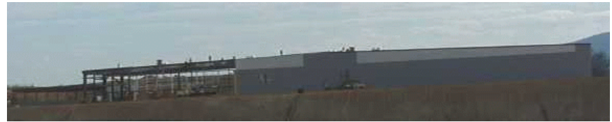
WTI construction progressing.
