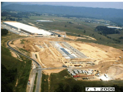
View of the Gatorade/Amcor sites as Amcor begins construction.
